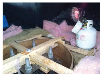
Innovation can be simple. PCL received the 2015 CCA Excellence in Innovation Award for replacing conventional heating and hoarding with ice-fishing tents and propane heaters when installing cast-in-place bored piles at the Heartland Substation project in Gibbons, Alta. The cost savings was \$415 per pile, or \$166,180, mainly due to savings on heating.
